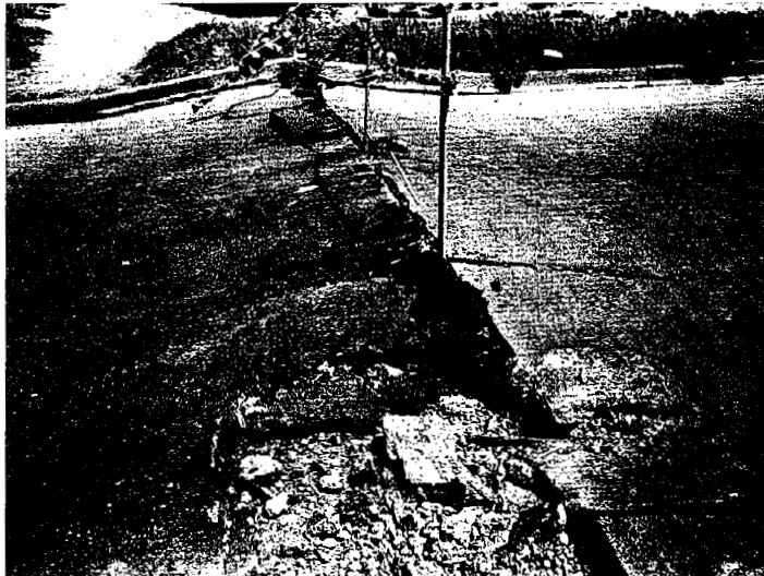
FIGURE 1 View of the deteriorated pavement at 600 Catamarca street, after the burst.
