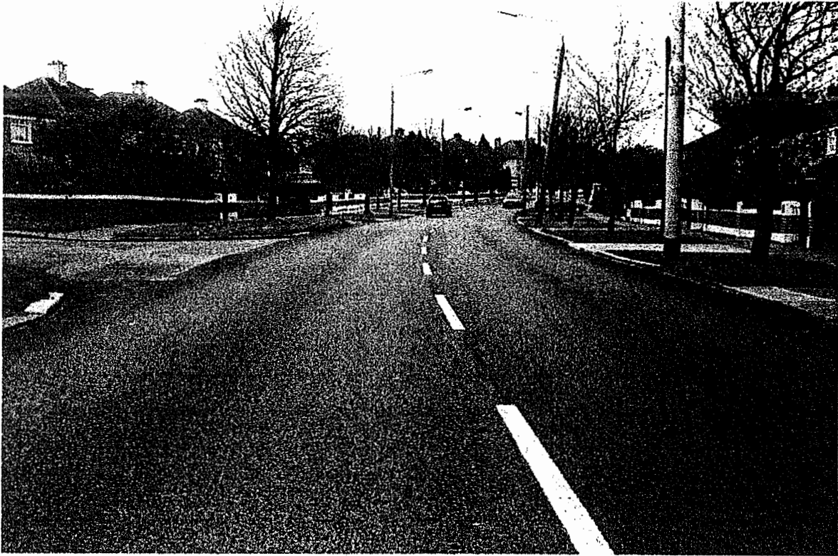
FIGURE 3 The Ballyroan Road after Resurfacing
