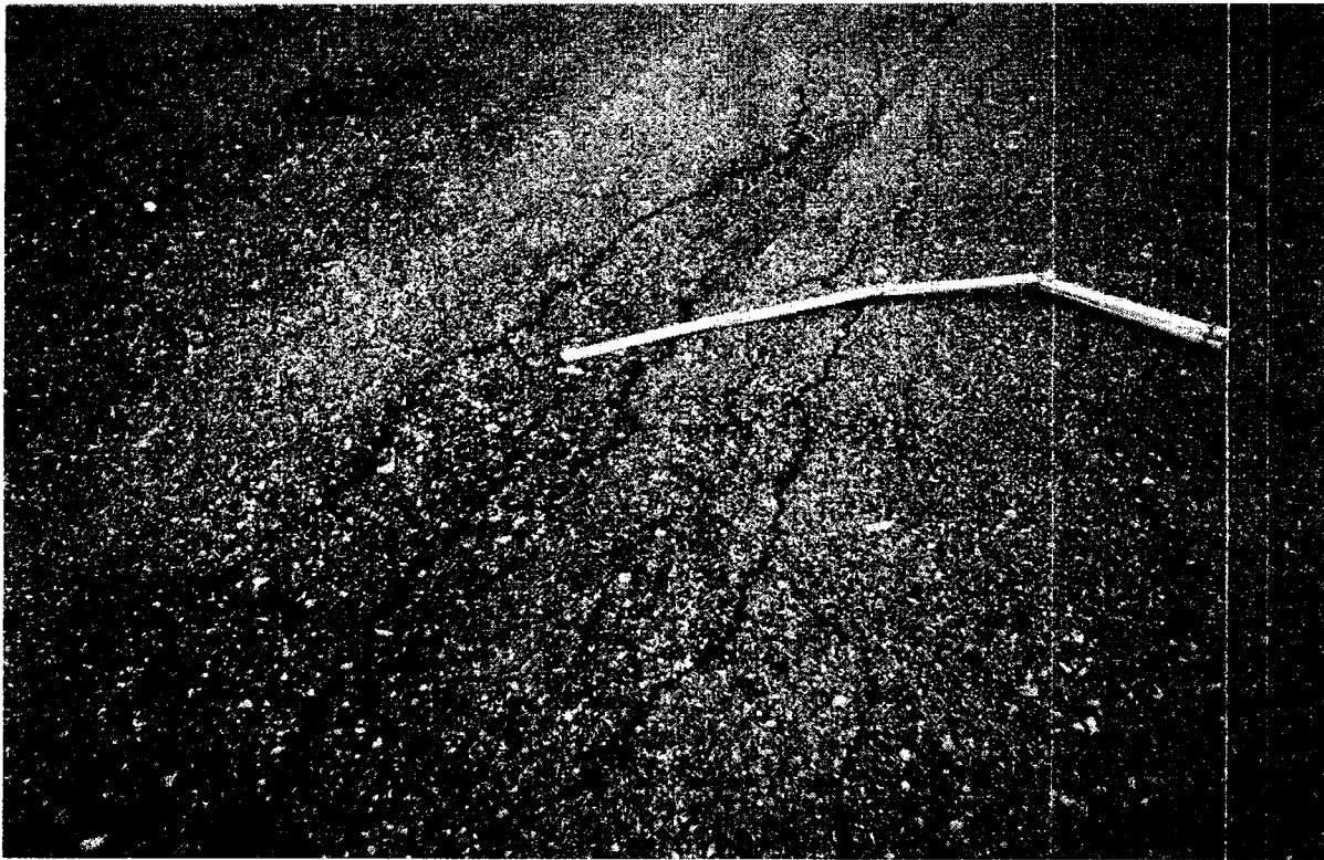
FIGURE 2 Typical pavement damage at Rhodes airport runway
