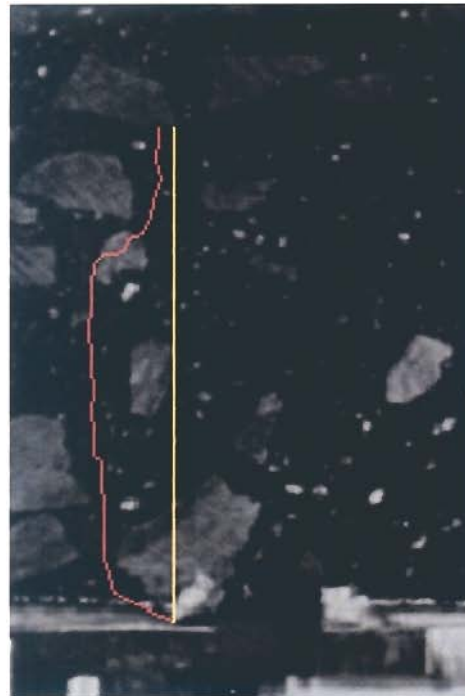
Color Plate II (See page 25, Plate 6) Electronically superimposed crack on unpainted beam – specimen HRA5HH1
